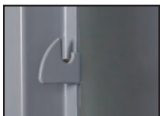
Main door latch hooks welded to frame
