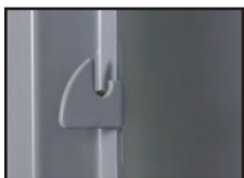
Main door latch hooks welded to frame
